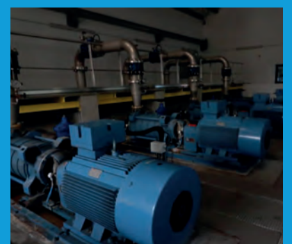
Station de pompage
